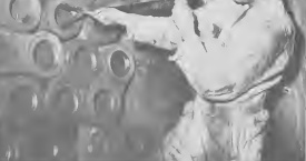
ALTHOUGH MUCH emphasis is placed on on-stream inspections, there is still work to do when a unit comes down. Measuring inner diameters of furnace tubes in L. Giel, above, and checking tube bundles, top left, is D. Henriquez. At left an inspector is hammer testing furnace tubes. MASKE HOGI enfasis ta worde poni ariba inspeccion mientras planta ta opera, ainda tin trabao di haci ora un planta baha. Midando diametro interior di tubonan di forno ta L. Giel, ariba, y controlando bundel di tubo, robet, ta D. Henriquez. Banda robet un inspector ta check tubo di forno.
